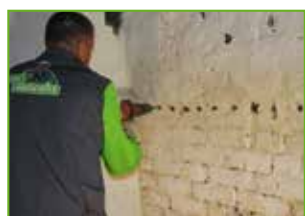
Horizontal drilling
